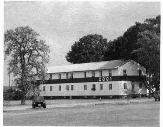
West end of the Original Armed Guard Gunnery School at Little Creek, Virginia of Oct. 15, 1941. (2001 Building)
